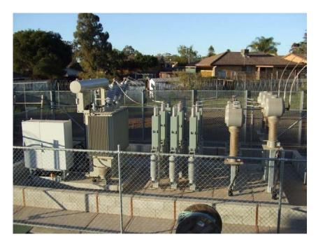
Figure 3.3: Ripple Injection Equipment at a Zone Substation (photograph courtesy of Essential Energy)
